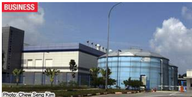
Intel Micron Flash Technologies wafer fabrication plant
